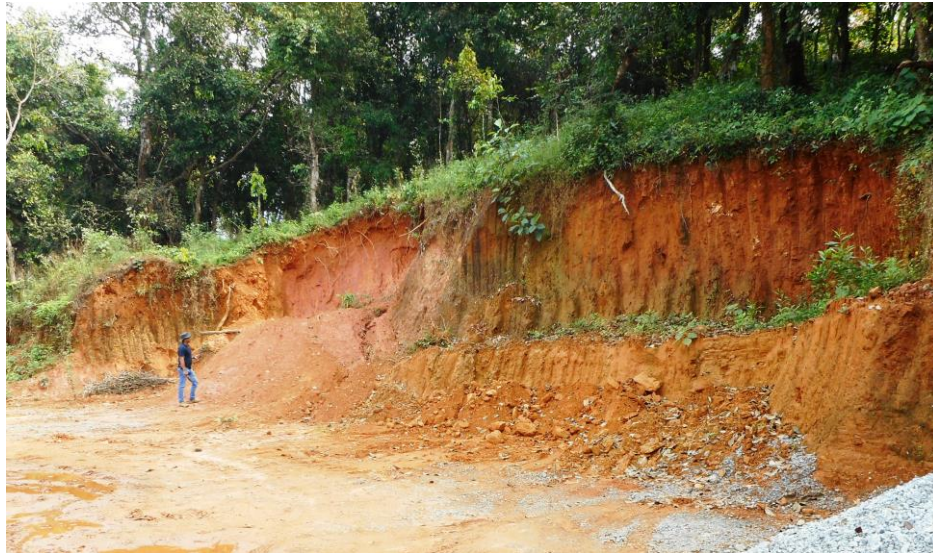
Photo 1: Extensive cut slope in in-situ soil between Kunetad and Panjali road section. TS O/4
