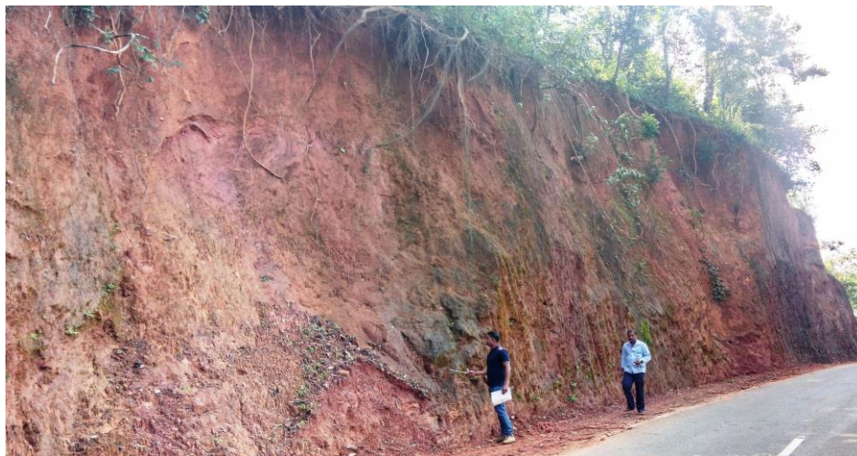
Photo 2: Extensive cut slope in soil along Solapur-Mangalore Highway (NH-13). TS O/3
