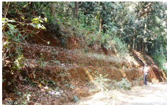
Photo 16: Benching of slope along Allallige – Hosmar road section. TS O/4
