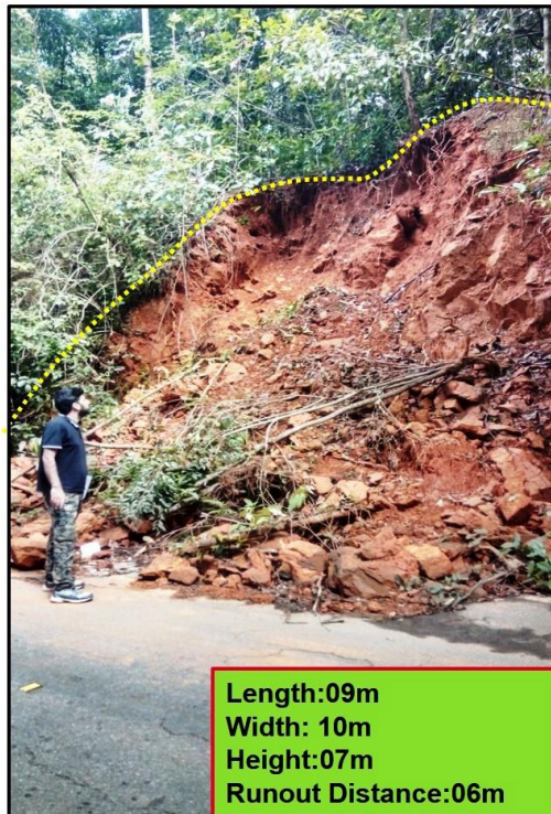
Photo 17: Cut slope/Slide along Mulluru - SK Border Road section (left) and Kerekatte - Harebail Road section (Right). TS O/3
