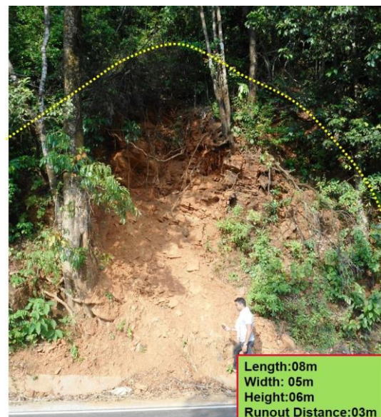
Photo 19: Landslide along Kundapur- Agumbe Road section. TS O/3
